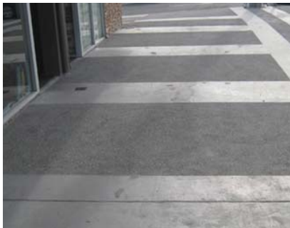
CONCRETE BANDING AND PLANTER - HEAVY SANDBLAST FINISH TO PROVIDE TEXTURE
