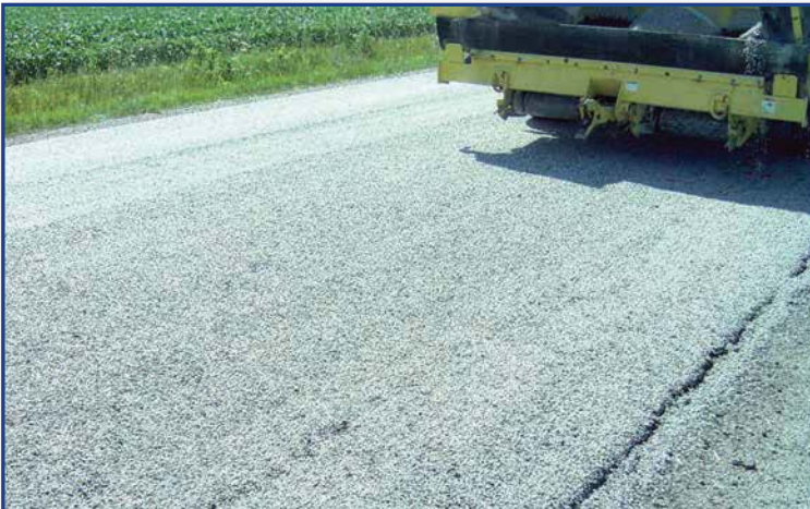
Aggregate protects FiberMat™ from traffic.
