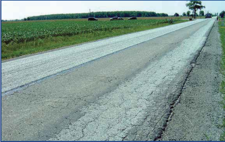
Existing cracked surface before FiberMat™.
