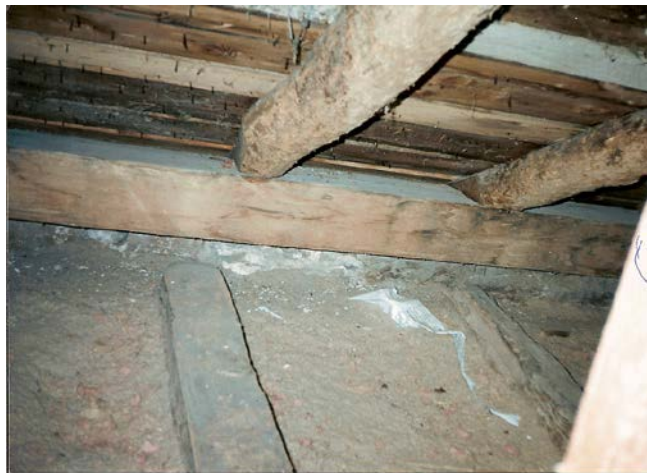
In the attic: note rafters dovetailed into plate
