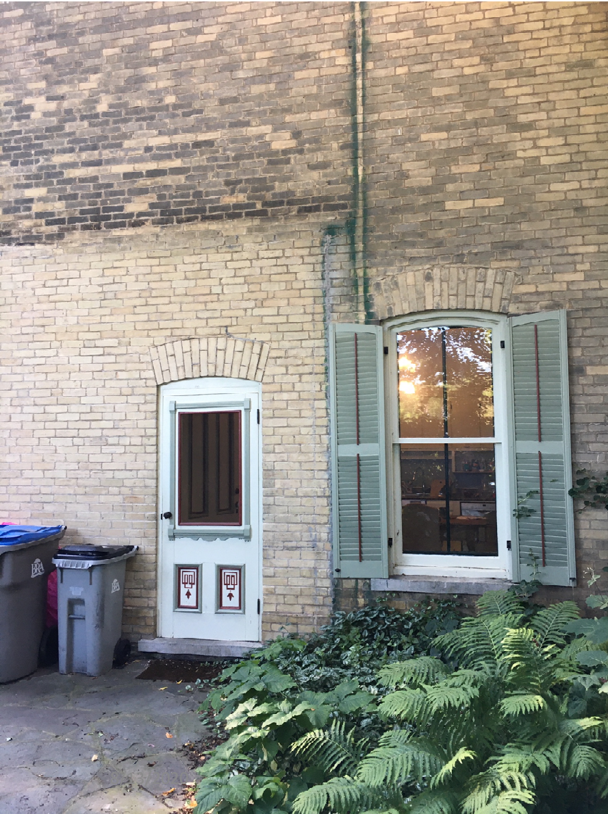
← Pic 1: north side of back of house – door to be converted to window – matching the existing window
