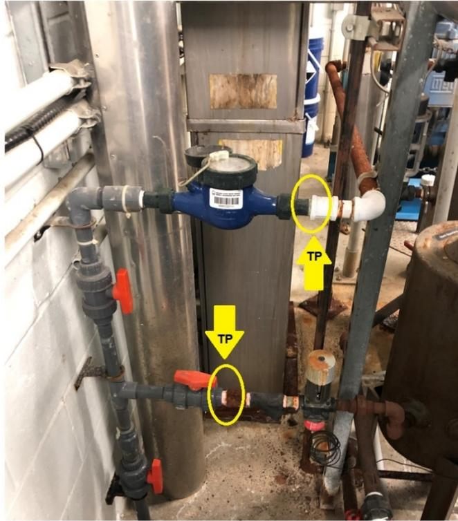
Figure 3 Tie in point associated with the soft water supply to the feedwater tank and to the blowdown receiver.
