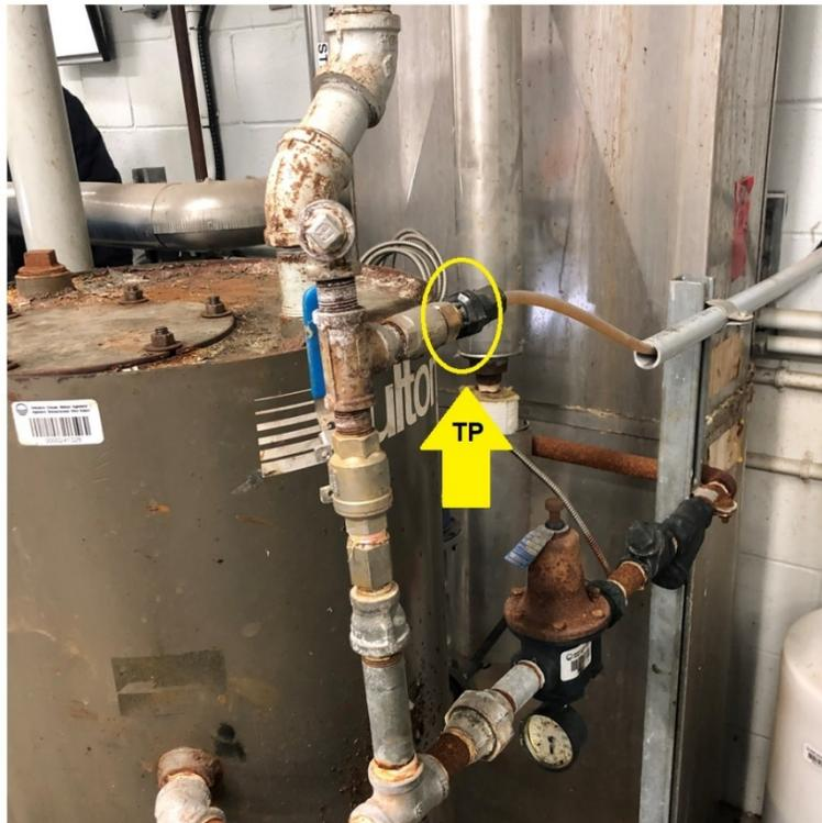
Figure 4 Tie in point of the chemical injection system associated with the feedwater tank.
